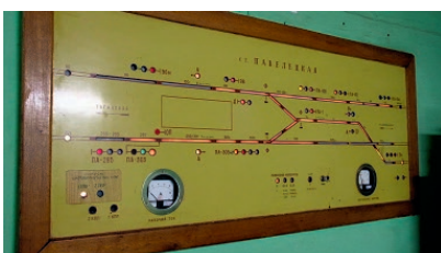
The track indicator with track layout mimic, operating console and relay equipment which were operated at the Paveletskaya station since 1954
