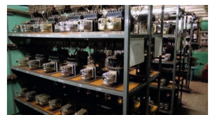
The track indicator with track layout mimic, operating console and relay equipment which were operated at the Paveletskaya station since 1954
