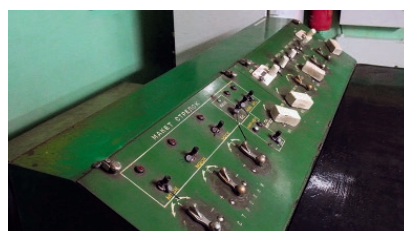
The track indicator with track layout mimic, operating console and relay equipment which were operated at the Paveletskaya station since 1954
