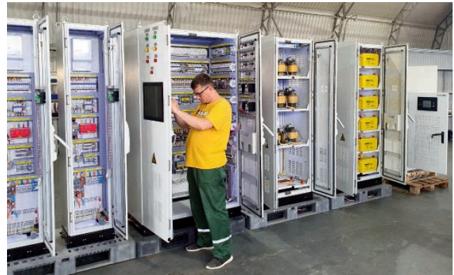
Installation of the UEP-U-M power supply unit
