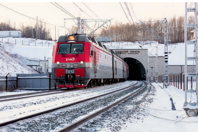
The Division’s signaling systems are used on the Trans-Siberian Railway section, which includes the brand-new Kerak tunnel
