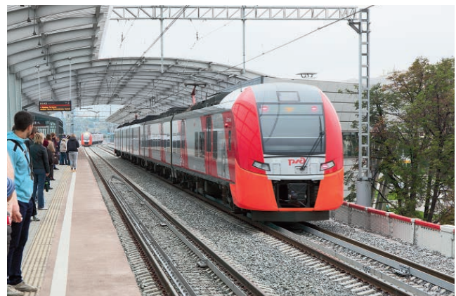
The Moscow Central Circle was equipped with computer-based interlocking systems by the Signaling Division of GC NPS
