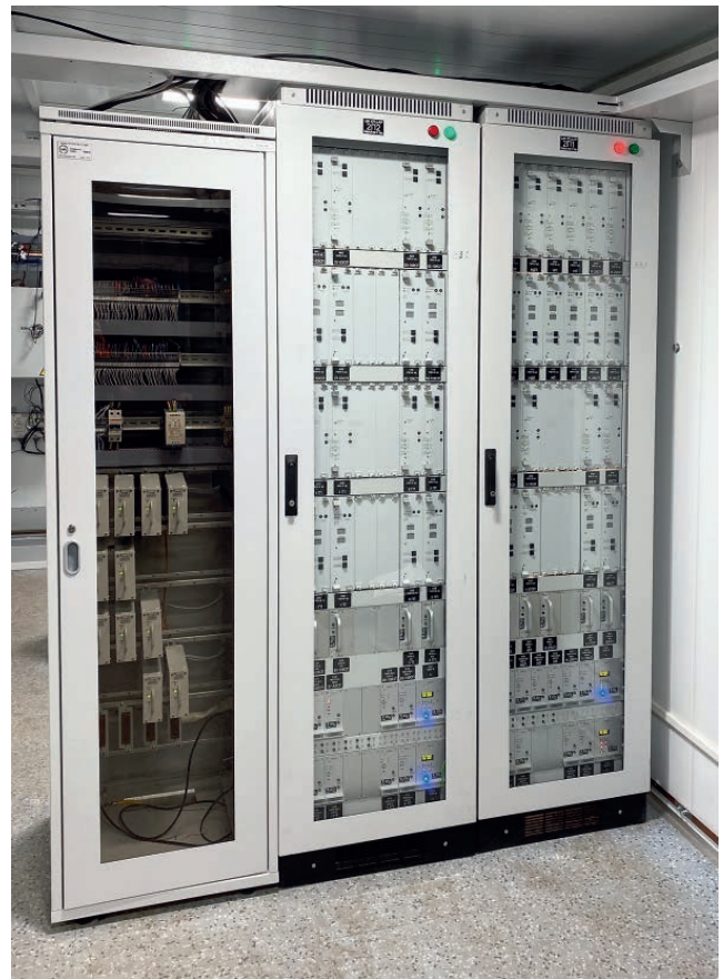
Digital track circuit monitoring module DM TCC-AR
